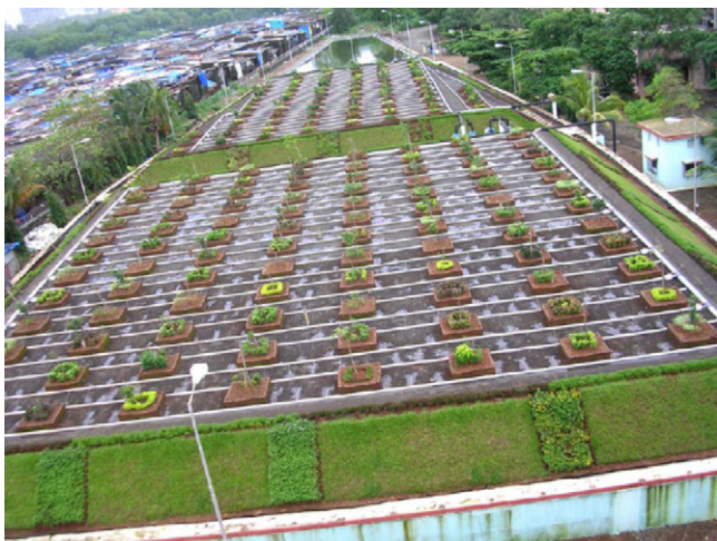
Fig. 6. Pictorial view of 3 million litres per day (MLD) sewage purification CSF plant at MCGM, Mumbai, India.
